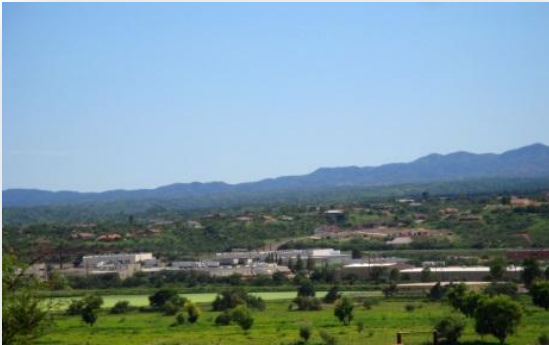
City of Nogales – Sewer Plant
