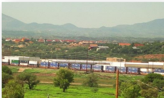
Railway behind Rio Rico Industrial Park
